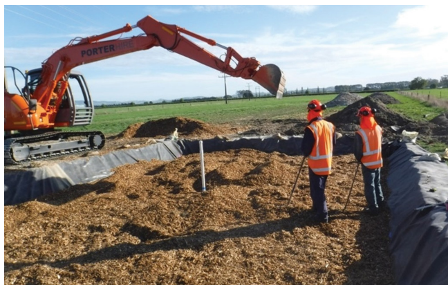
Installing a wood-chip bioreactor (Lincoln Agritech image)
