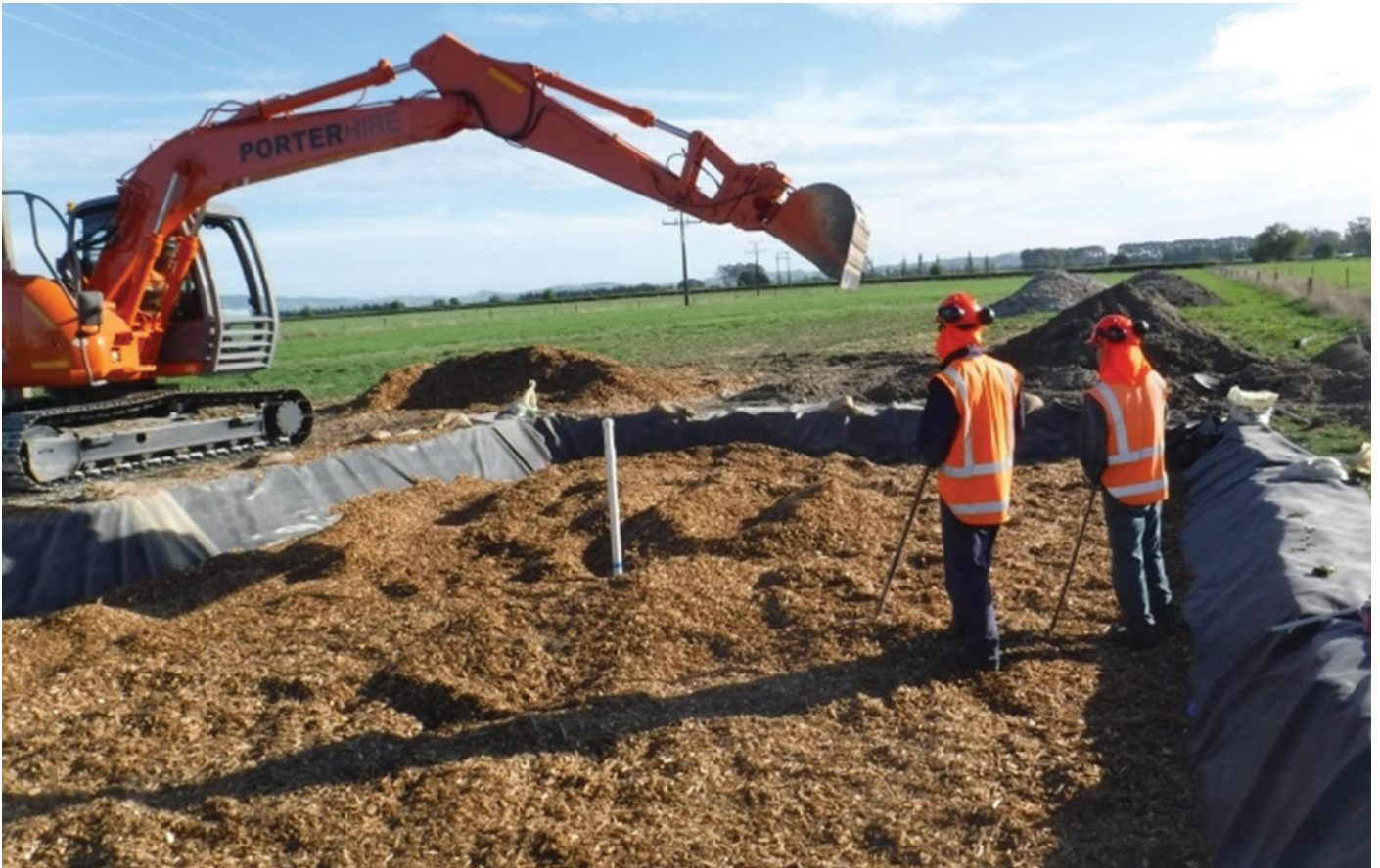
Installing a wood-chip bioreactor (Lincoln Agritech image)
